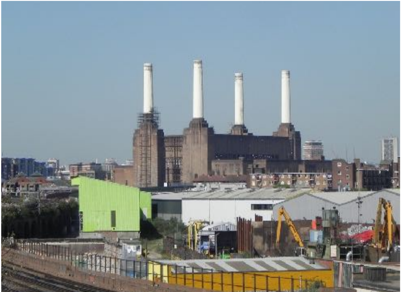
View from Wandsworth Road rail station overbridge.
